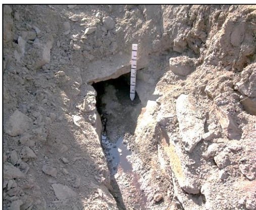
Aqueduc souterrain, cliché H. Pigeyre
